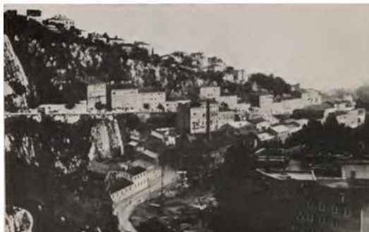
Plate 82. Sušak: valley of the Fiume Eneo The photograph looks southwards from the Sušak-Delnice road. The building with the tall chimney in the centre foreground is a rice-mill.
