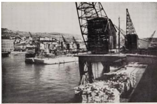
Plate 80. Sušak: Gat E. Bačića, looking east-north-east from Gat Aleksandra I The three cranes seen on the north side of Gat E. Bačića are of the electric (traveling) portal type with a capacity of 1½ tons each; those on Gat Aleksandra I have the same capacity but are of the semi-portal type.
